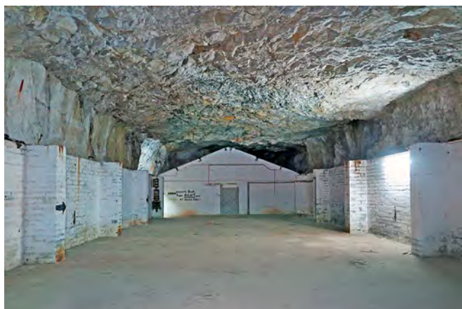
Arow Street: the remains of a truss-roofed building. Photo Clive Penfold
